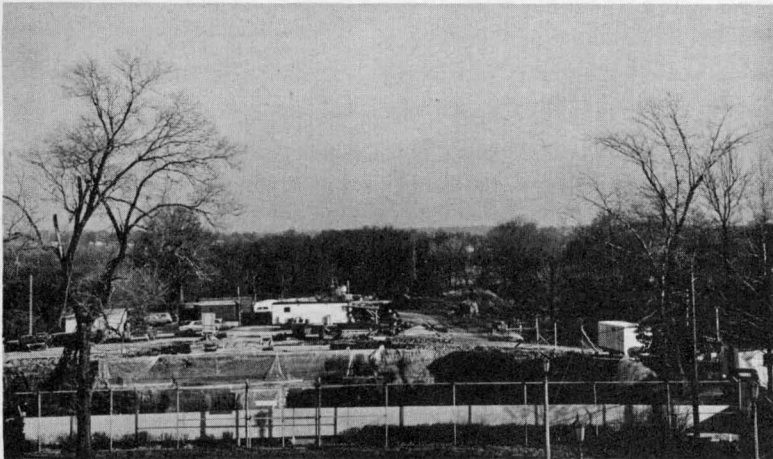
Construction work begins on Math and Modern Languages Building
